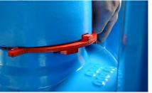
During installation, the correct alignment of the notches must be ensured (see photo).
