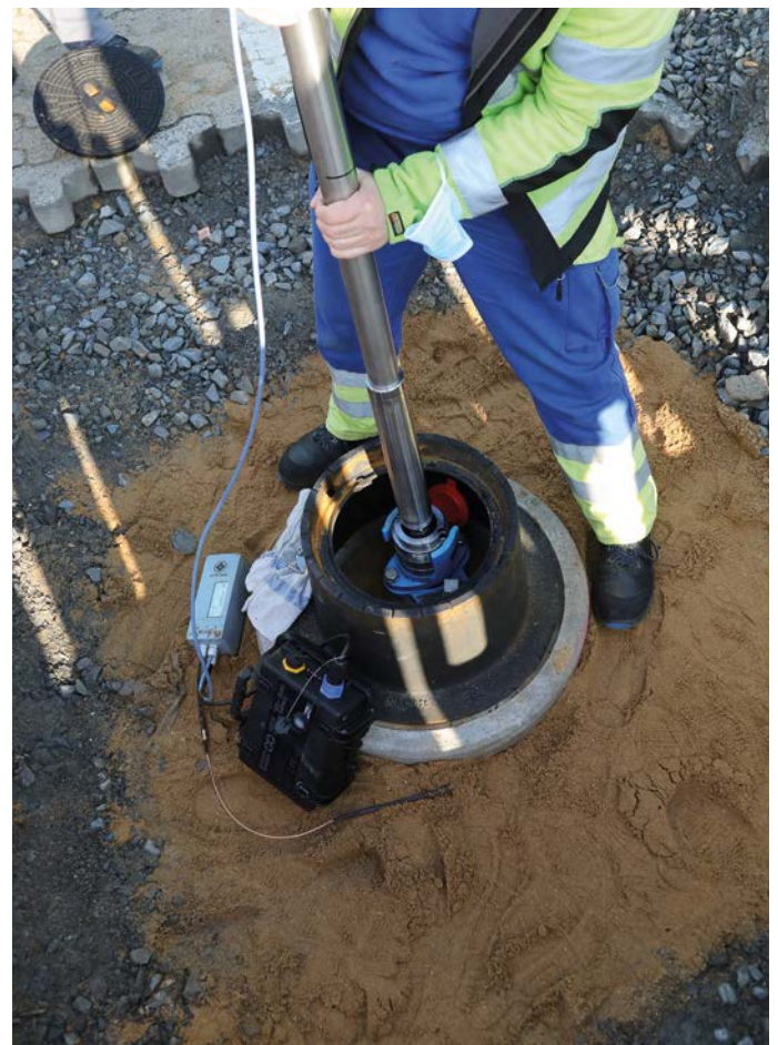
Trial installation of measurement lock
