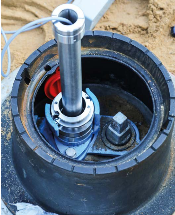
Trial installation of measurement lock
