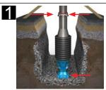
Establish a foundation for the hydrant base in the trench.
